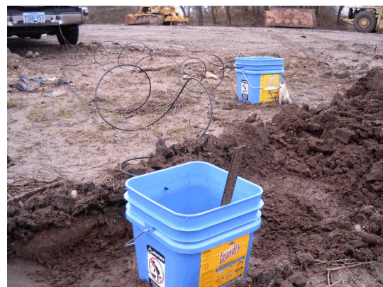
CES will perform infiltration tests at the Site
