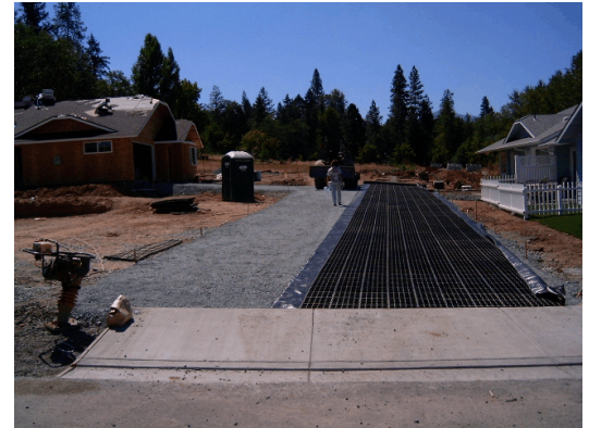
Partial installation of StabiliGrid in Horizon Village. 8-24-06.
