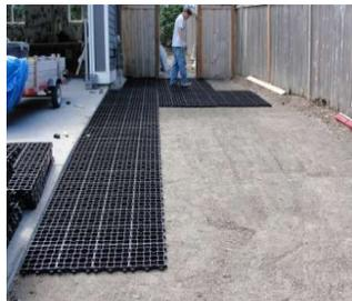
**Step1:** We've already saved you some work. 12 Individual grids are pre-connected in easy-to-install units. This means you may install 12 grids at a time.
