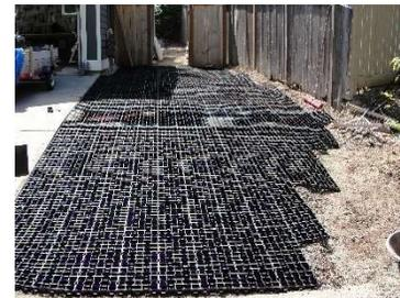
**Step4: Done in a flash!** - the grids are locked into place and anchored. This rules out the possibility of raised edges or migration.
