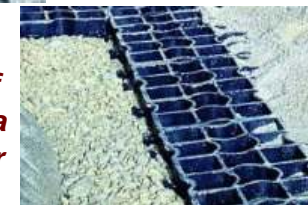
Clean washed coarse sand, buckshot or gravel may be used for a top footing layer, from 3/4" to 1 1/2" deep or more.
