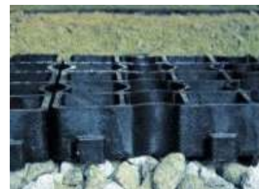
A thin layer of gravel may be required beneath the grids.
