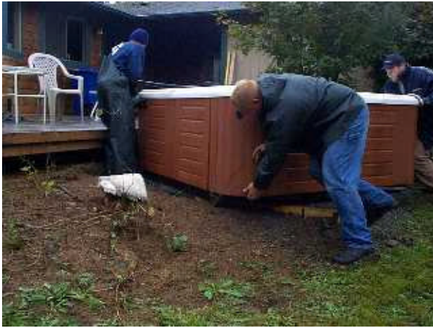
Installing the hot tub on the base - app. 5 minutes.
