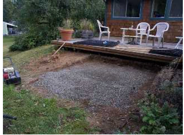
Overview of the hot tub installation pad area.
