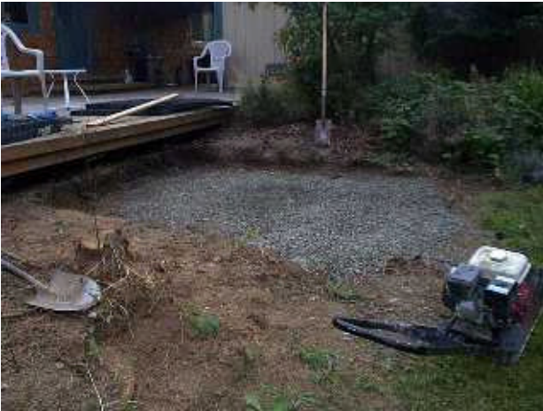
Minimal leveling layer of porous gravel is compacted.
