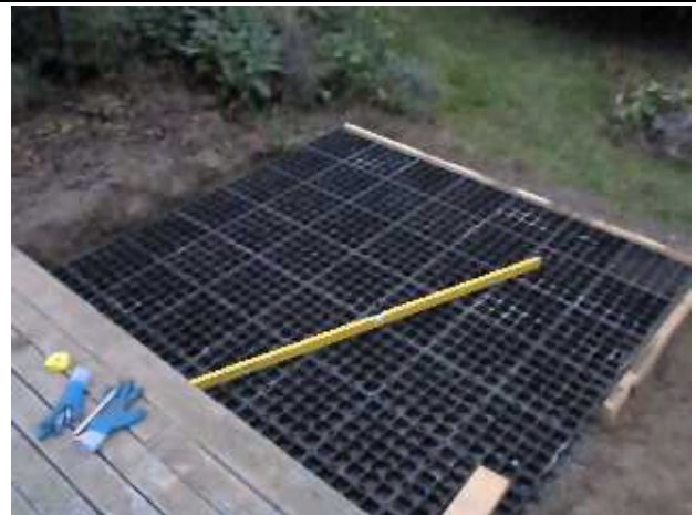
Overhead view of the outdoor hot tub base.
