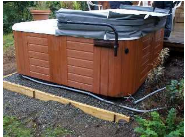
Installing the cover for the exterior hot tub.
