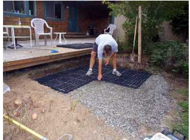
StabiliGrid™ pervious pavers installed - app. 3 minutes.
