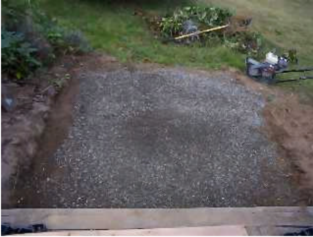
Ground is graded level.
