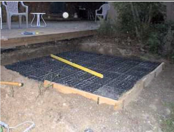
Confirm the hot tub pad is level.
